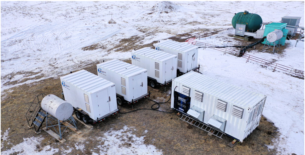
A site owned and operated by Brox and leased by PermianChain to run one of our 300kW data centres to power 96 ASIC miners.
